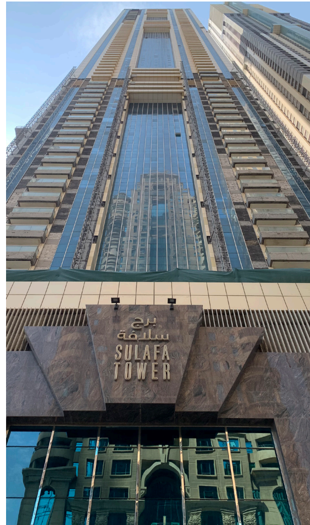
Sulafa Tower, Dubai / UAE
