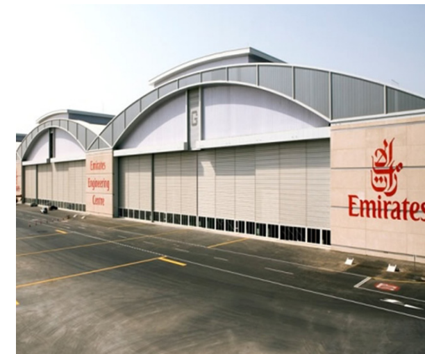
Emirates Airlines A380 Maintenance Hangars Steel Roof, Dubai / UAE
